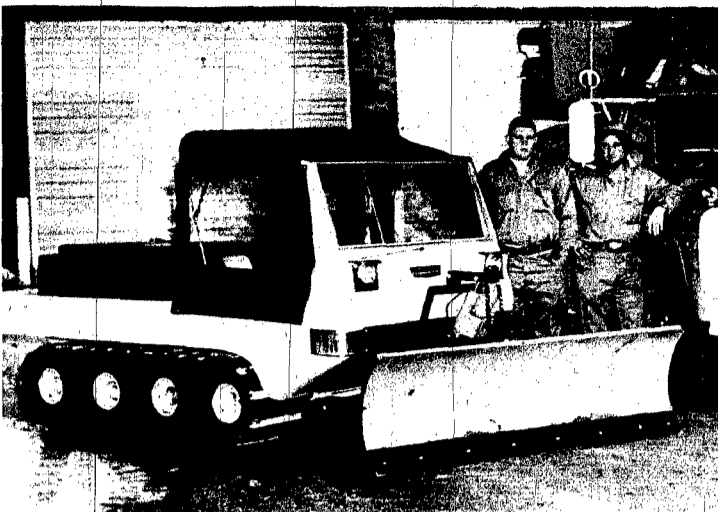
NEW EQUIPMENT for Wayne County Public Power District is shown by Dean Bruggeman (left) and Ros Reiter. The truck-vehicle is a "Categorator" which can travel in rural areas before roads are open. The new hydraulic hole digger for poles is on the truck on the right.
